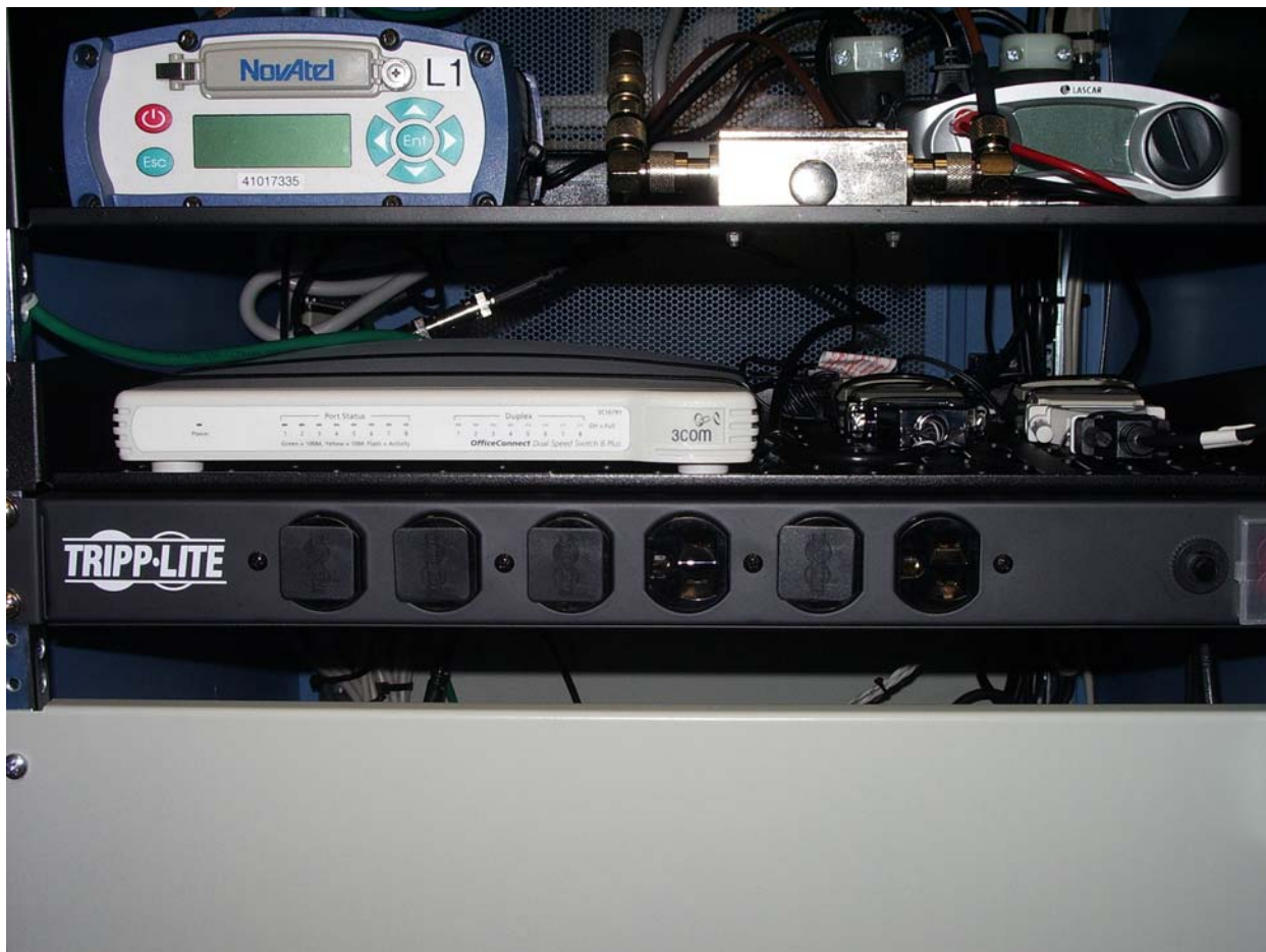
Rack Interior, Front (Top to Bottom: GPS Shelf, Network Shelf, Un-UPSed Power Strip)
