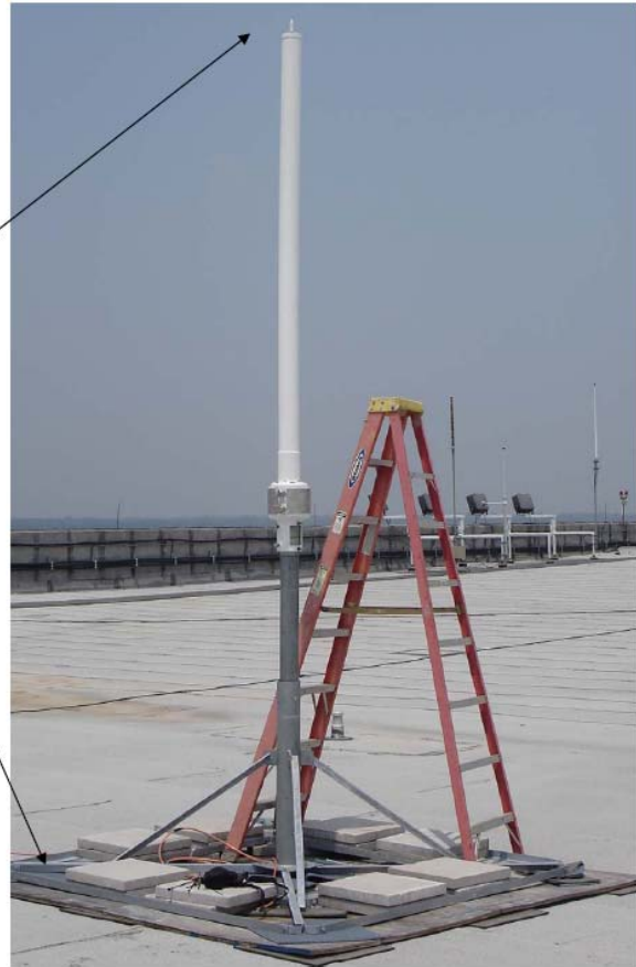
IAH FAA GBPM, GPS Antenna/Ballast Mount Representation and Details
