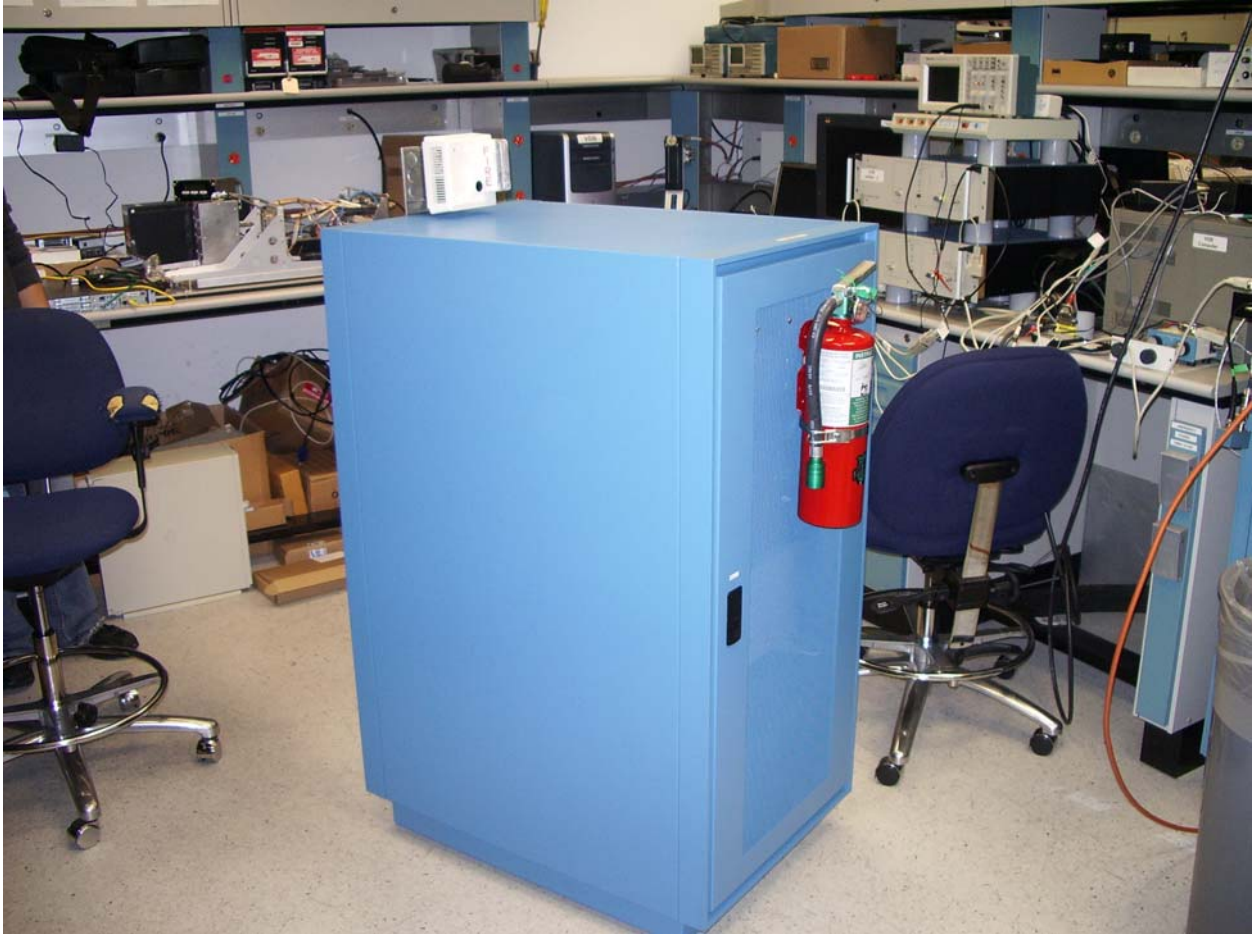
Rack Exterior (Front: Fire Extinguisher Door, Rear: Fire Sensor Door)
